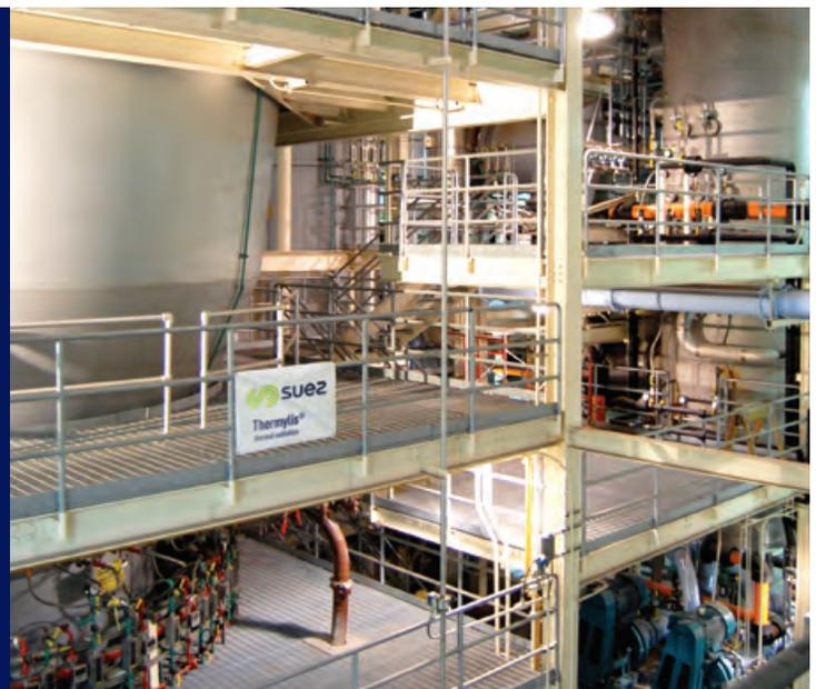
the combustion. The “three T’s” - turbulence, time, and temperature - make fluid bed incineration the most economical and environmentally sound method of sludge disposal. Uniform bed temperature, the result of steady turbulence, simplifies PLC/PC automation and logic control systems. Data gathering for compliance reports becomes much easier.
