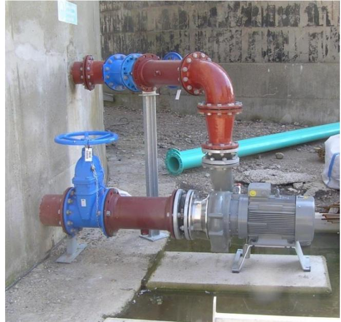
**Figure 3: Monsal ADT Pump Mixing Installation**
