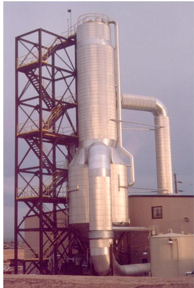
**Figure 5: Typical Vertical Tube Falling Film RCC\* Vapor Compressor Evaporative System**
