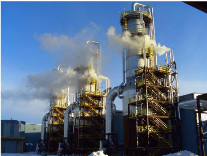
Figure 5: 3,000 gpm Produced Water Evaporator System at Suncor Firebag Stage 2
