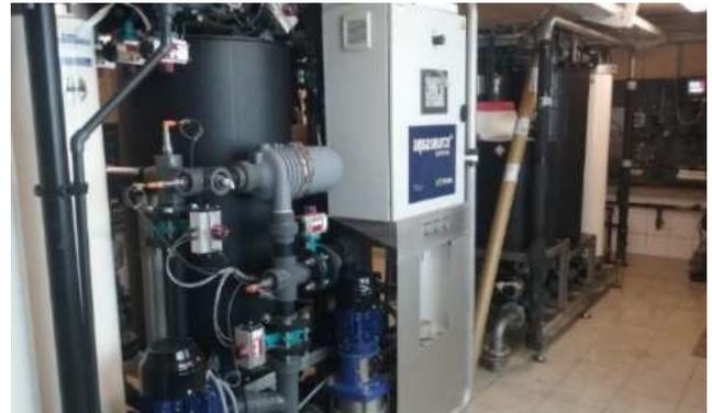
Figure 1: The two aquasource\*Z-XS on site
