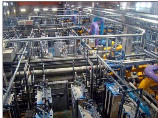
Figure 1: EDR water treatment plant at ATLL
