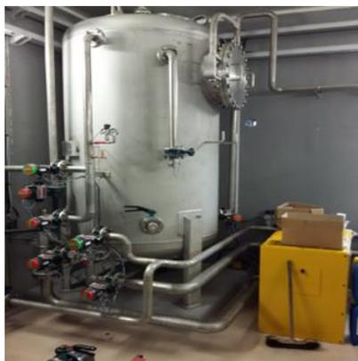
**Figure 1: Granular Activated Carbon**
