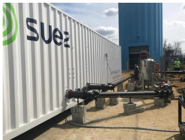
**Figure 1: SUEZ specialty ion Exchange container used to remove PFAS in the drinking water supply**
