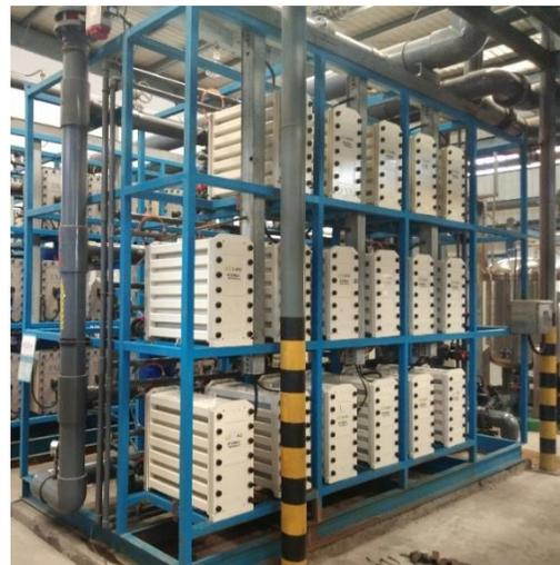
Figure 1: E-Cell MK-7 installation at customer site
