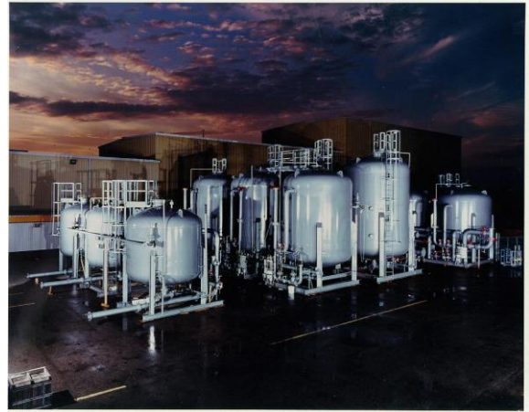
Figure 4: Tanks at the Manufacturing Plant.
